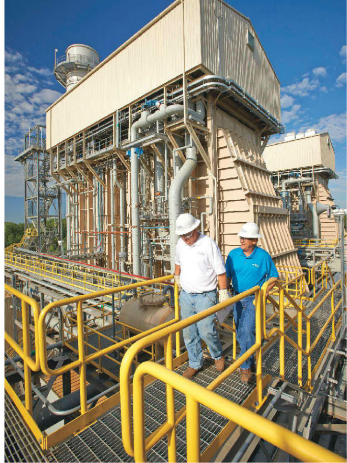
Facilities such as Duke Energy's 620-megawatt Buck Combined Cycle Station in Rowan County combine gas combustion turbines and steam turbines to convert natural gas to electricity.
